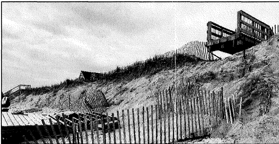
Figure 1: Photograph of Beach Access-8 being dismantled.
