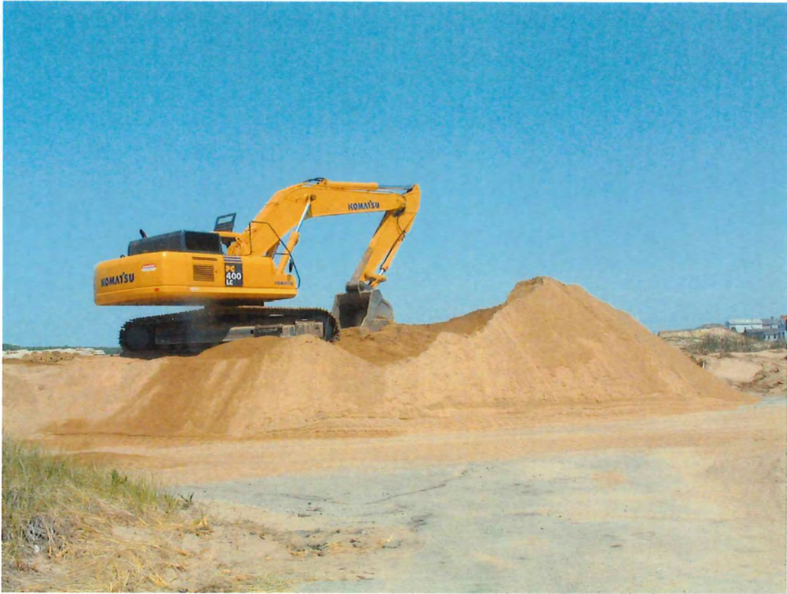
PHOTOGRAPH 1: DAY 4, STOCKPILING OF NEW SAND BEHIND DCR BUILDING.
