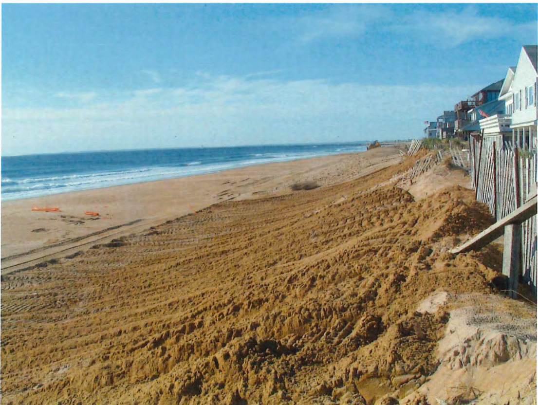
PHOTOGRAPH 2: NEW SAND ADDED TO NORTHERN END OF DUNE UP TO PUBLIC ACCESS #2.
