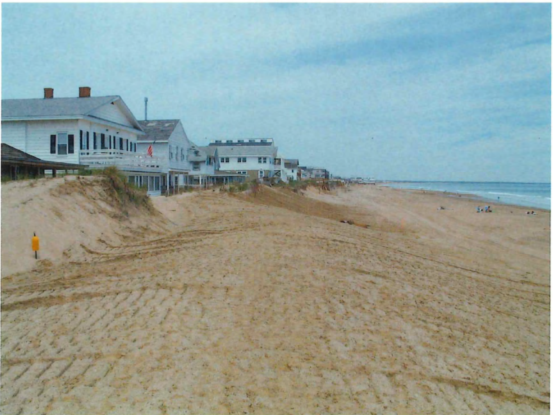
PHOTOGRAPH 8: THE NORTHERN END OF THE COMPLETED DUNE WITH ADDED SAND UP TO PUBLIC ACCESS #2.
