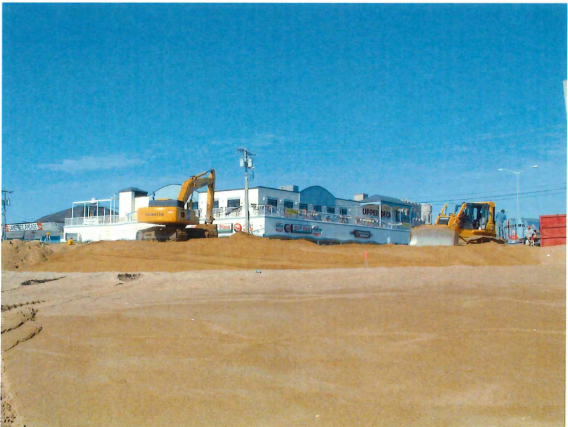
PHOTOGRAPH 12: SAND IS FORMED INTO THE PROPOSED DUNE AT THE END OF BROADWAY ST.
