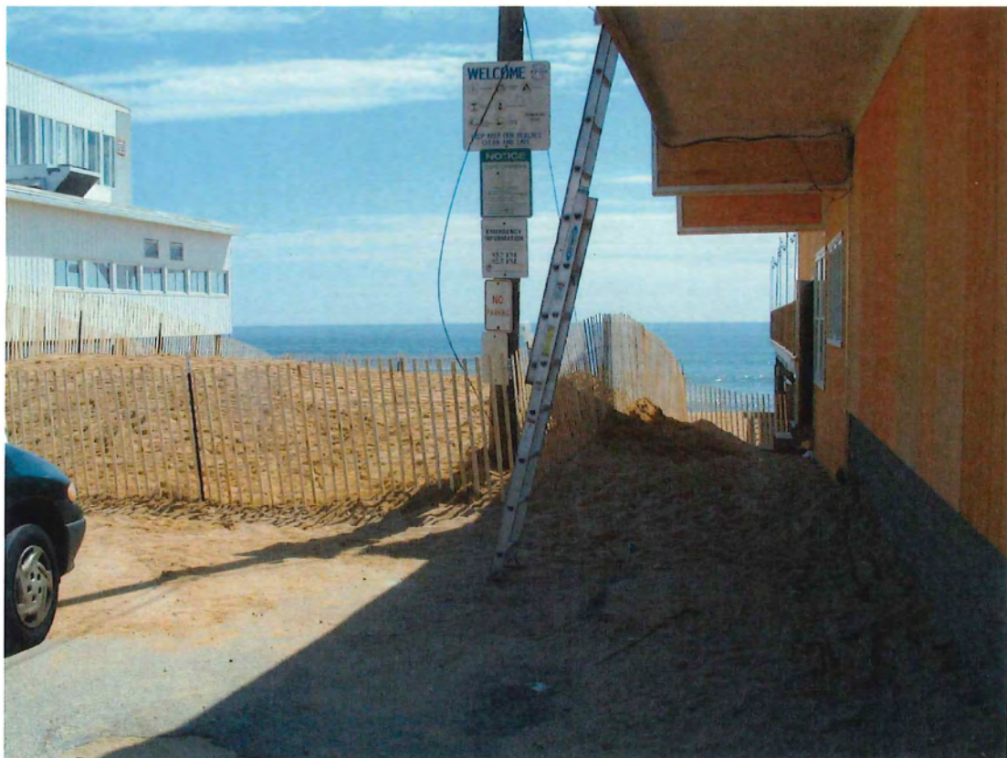
PHOTOGRAPH 22: THE COMPLETED DUNE BETWEEN BUILDINGS WITH ACCESS TO THE BUILDING.
