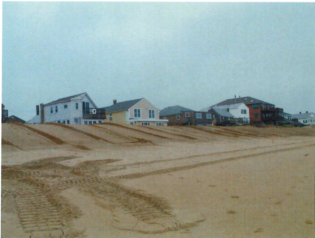
PHOTOGRAPH 12: THE NORTHERN END OF THE PROPOSED DUNE IS COMPLETED AS OF JUNE 5, 2007, DAY 8.
