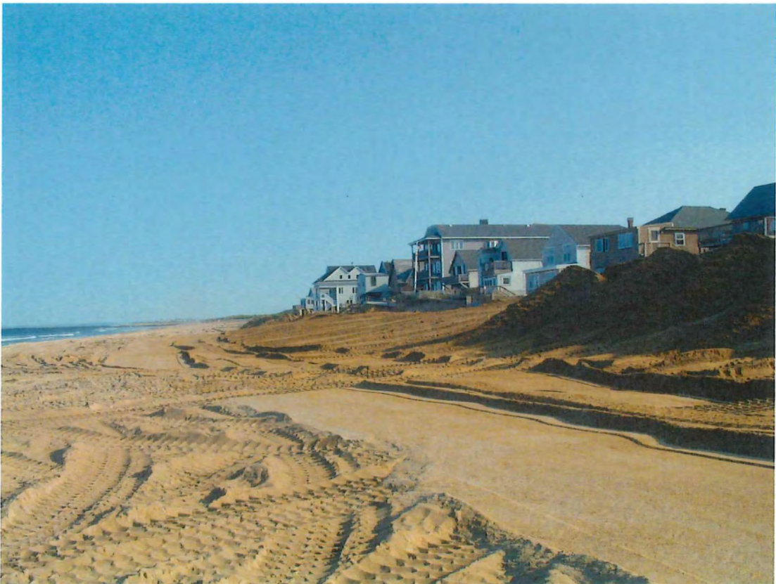
PHOTOGRAPH 4: SHAPING OF PROPOSED DUNE.
