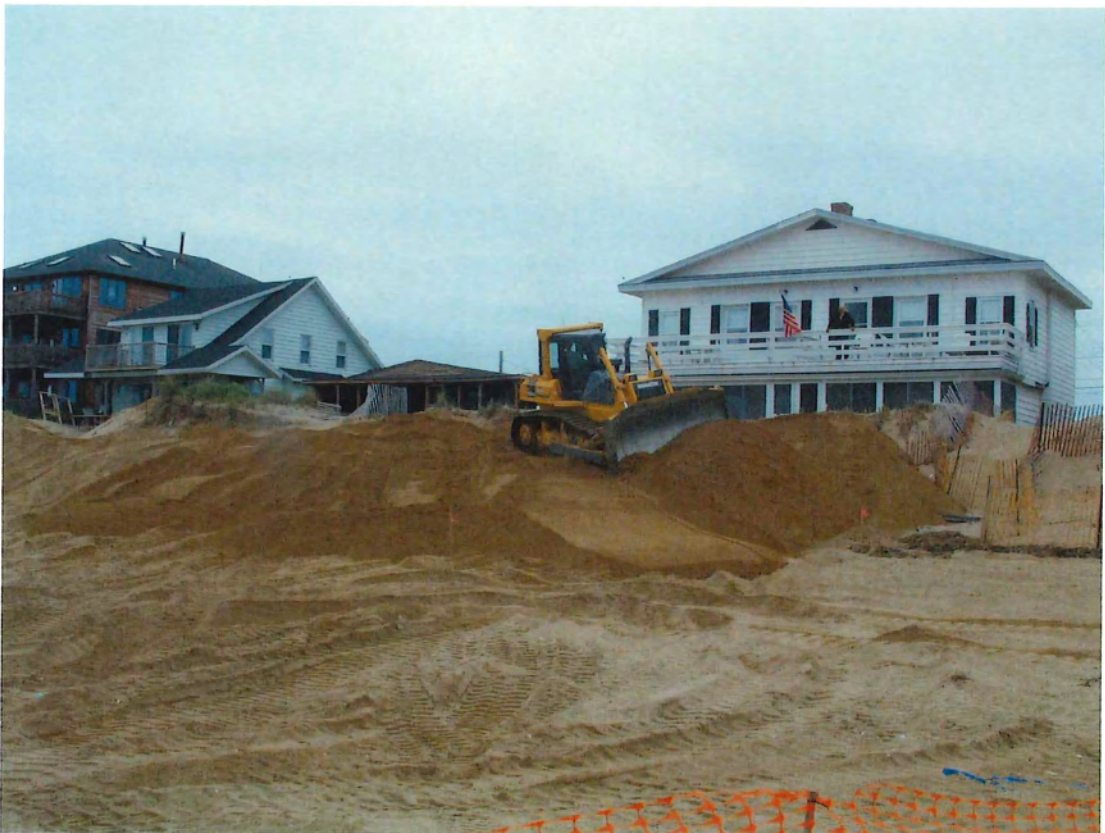
PHOTOGRAPH 6: SHAPING THE TRANSITION INTO THE EXISTING DUNE.
