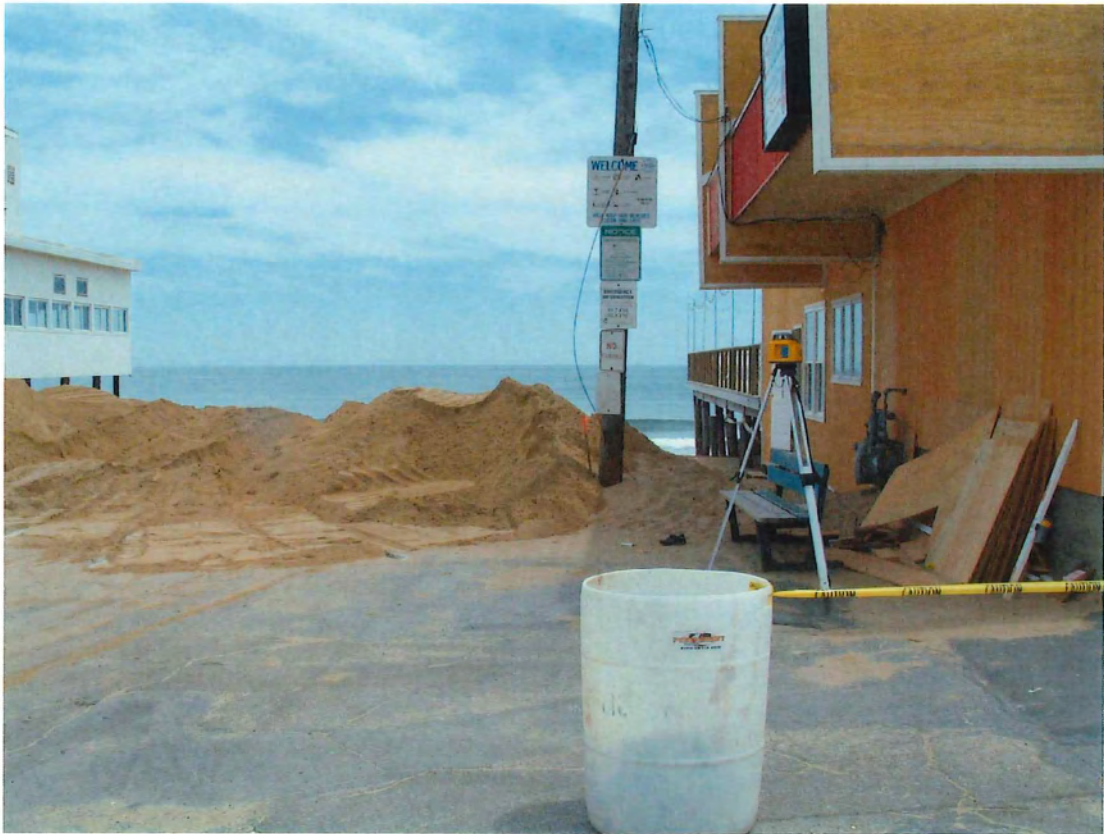
PHOTOGRAPH 15: THE PROPOSED DUNE TAKING SHAPE BETWEEN THE BUILDINGS.
