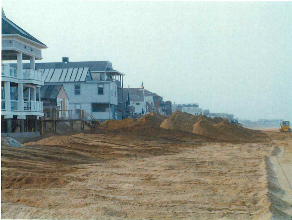
PHOTOGRAPH 11: NEW SAND HAS BEEN GRADED TO MAKE ROOM FOR MORE.
