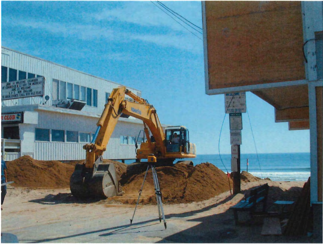
PHOTOGRAPH 13: SAND BEING FORMED INTO THE PROPOSED DUNE IN BETWEEN BUILDINGS.
