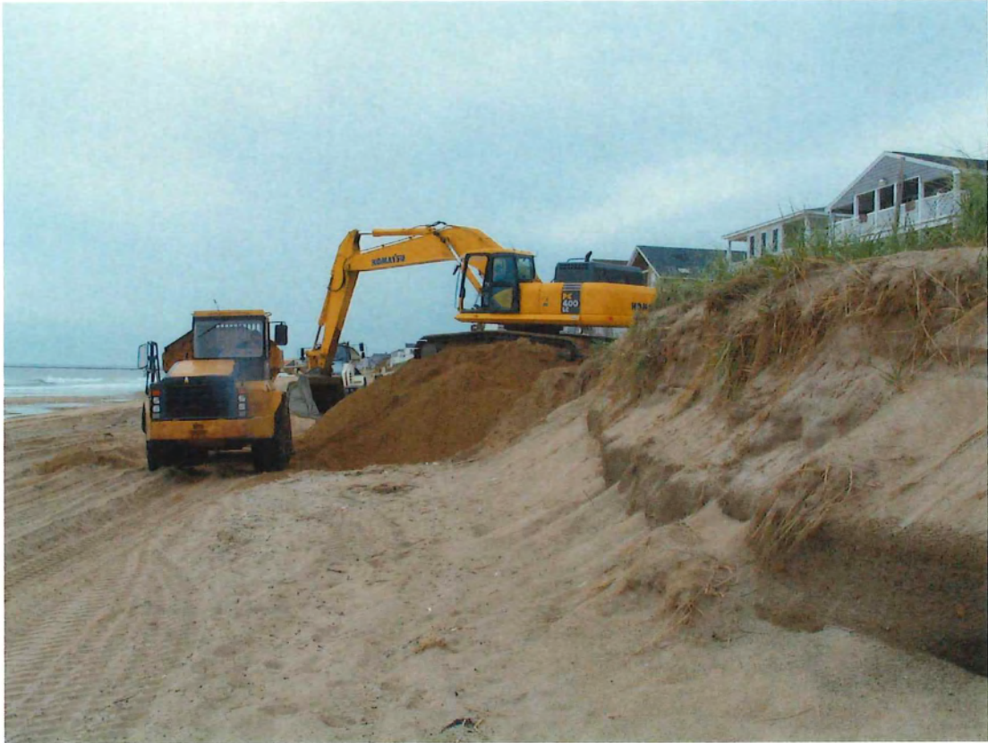
PHOTOGRAPH 5: STOCKPILE AND LOADING AREA AT PUBLIC ACCESS #4.
