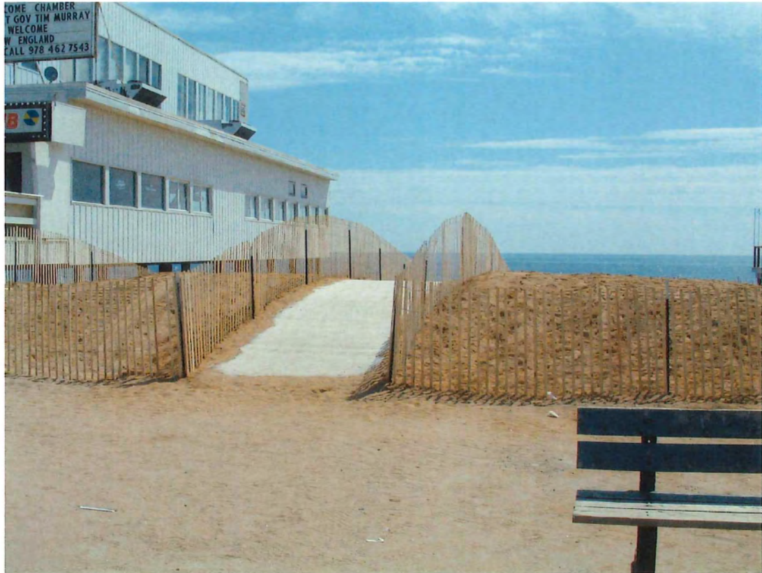
PHOTOGRAPH 23: THE COMPLETED DUNE BETWEEN THE BUILDINGS WITH SNOW FENCE AND MOBI-MAT.
