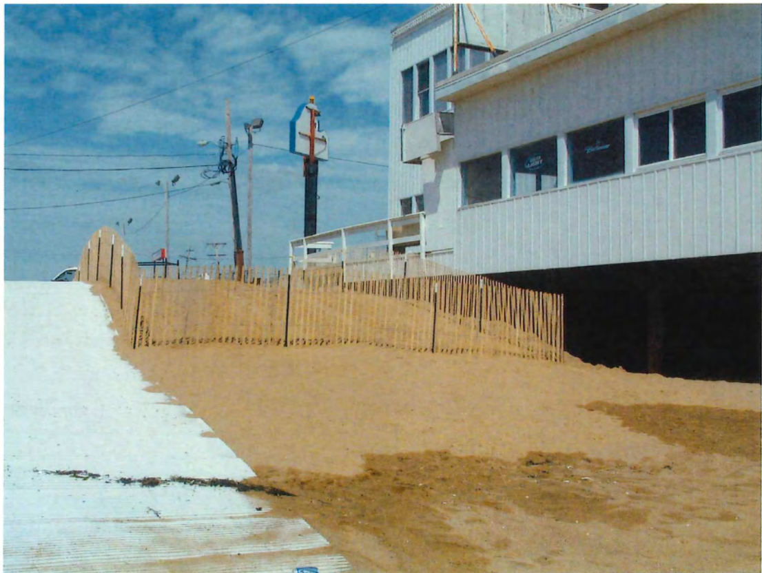
PHOTOGRAPH 24: THE COMPLETED DUNE BETWEEN THE BUILDINGS WITH SNOW FENCE AND MOBI-MAT.
