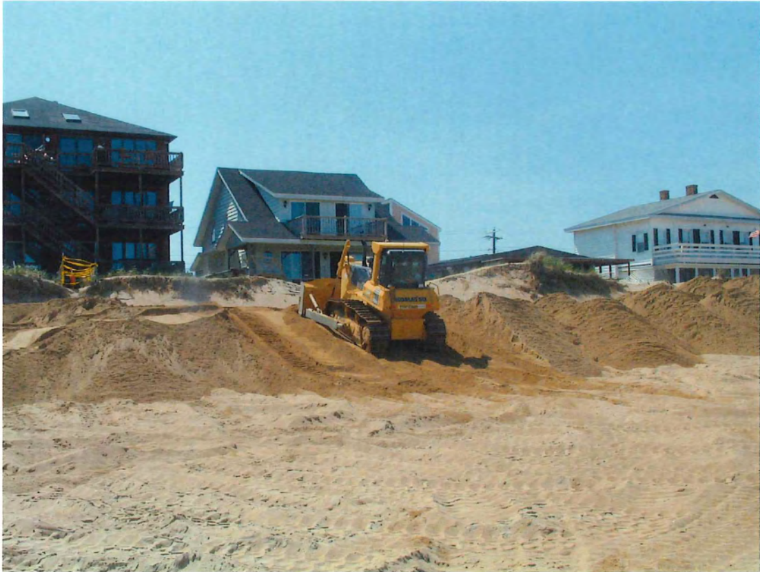
PHOTOGRAPH 3: BEGINNING TO FORM THE PROPOSED DUNE.
