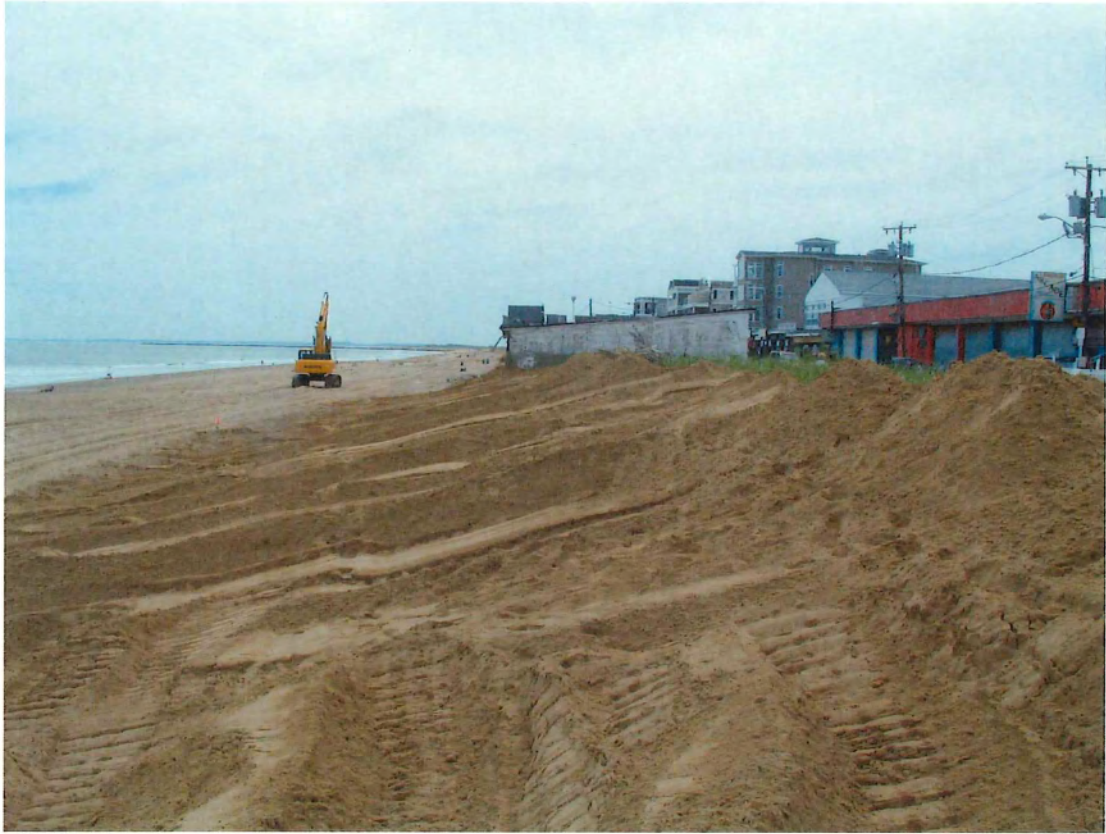
PHOTOGRAPH 11: NEW SAND IN FRONT OF EXISTING SACRIFICIAL DUNE BEGINNING TO TAKE SHAPE.
