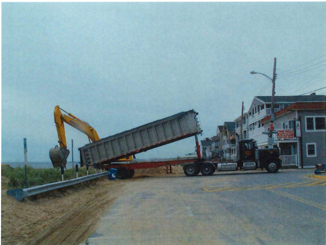
PHOTOGRAPH 4: NEW SAND BEING DELIVERED AT PUBLIC ACCESS #4.
