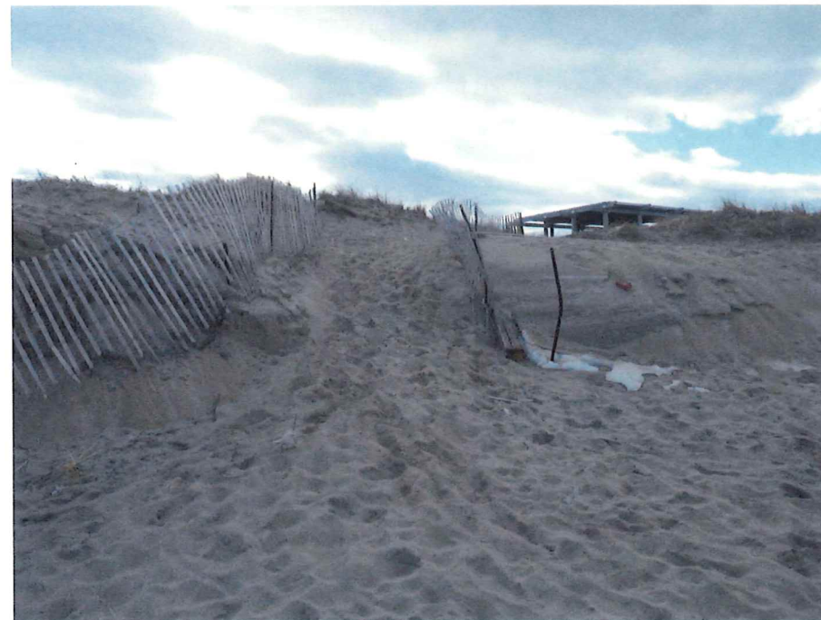
PHOTOGRAPH 8 Reservation Access No. 4
