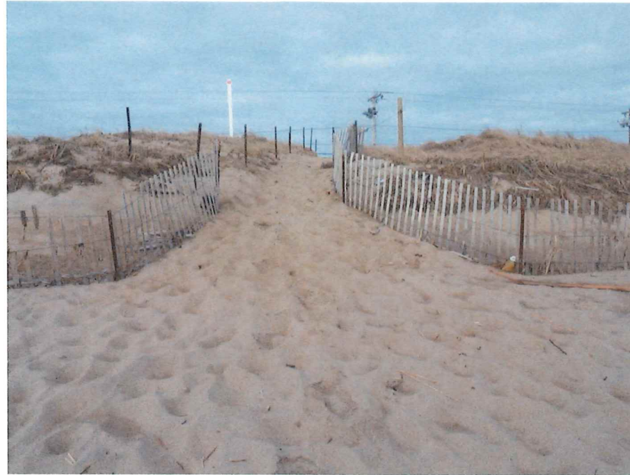
PHOTOGRAPH 29 Salisbury Beach Public Access No. 13 (Beacon Street)
