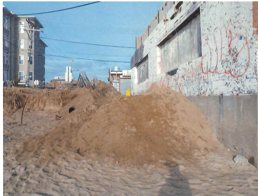
PHOTOGRAPH 16 Ocean Front S. Dune Crossing No. 4 (South side of building)
