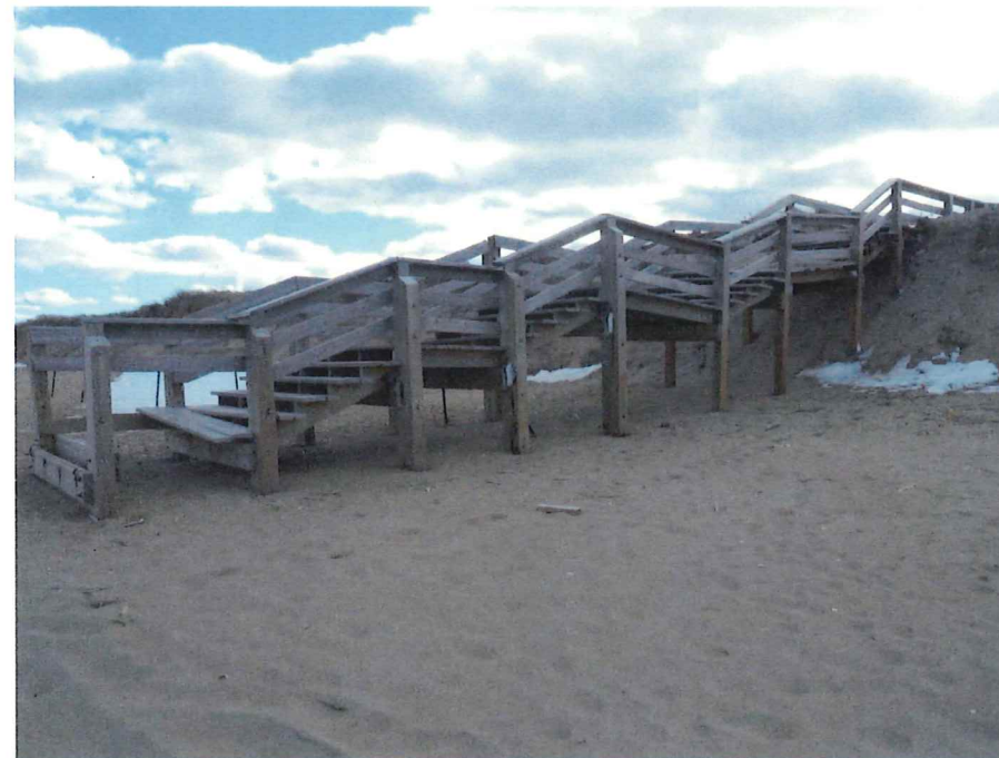
PHOTOGRAPH 6 Reservation Access No. 2
