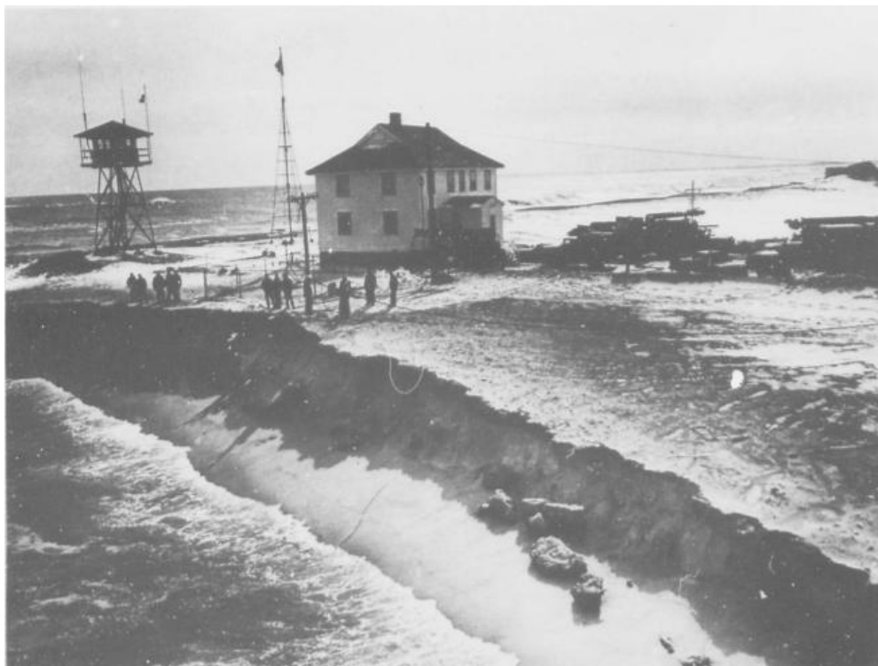
Figure 2.4. Shear erosion from February winter storm of 1969, when the Coast Guard building still sat near the jetty. Reservation Terrace, MA (photo from Boston Globe).
